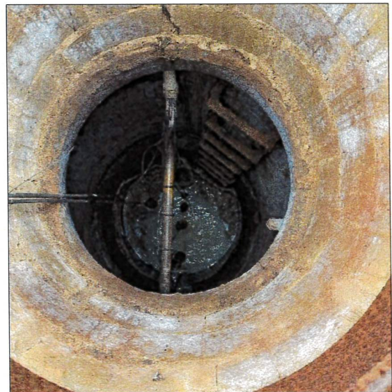
Figure 2 – Highway Lift Station Wet Well
